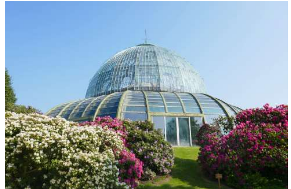
For instance, the Royal Greenhouses in Brussels are heated by the local WtE plant.
